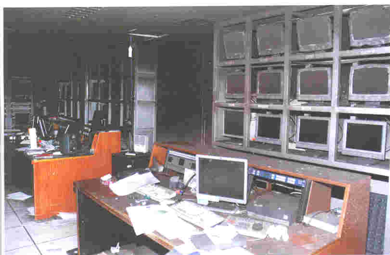
Most of the broadcasting machines were damaged after the attack
