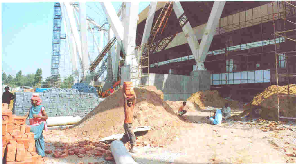
The Commonwealth Games National Stadium under construction
