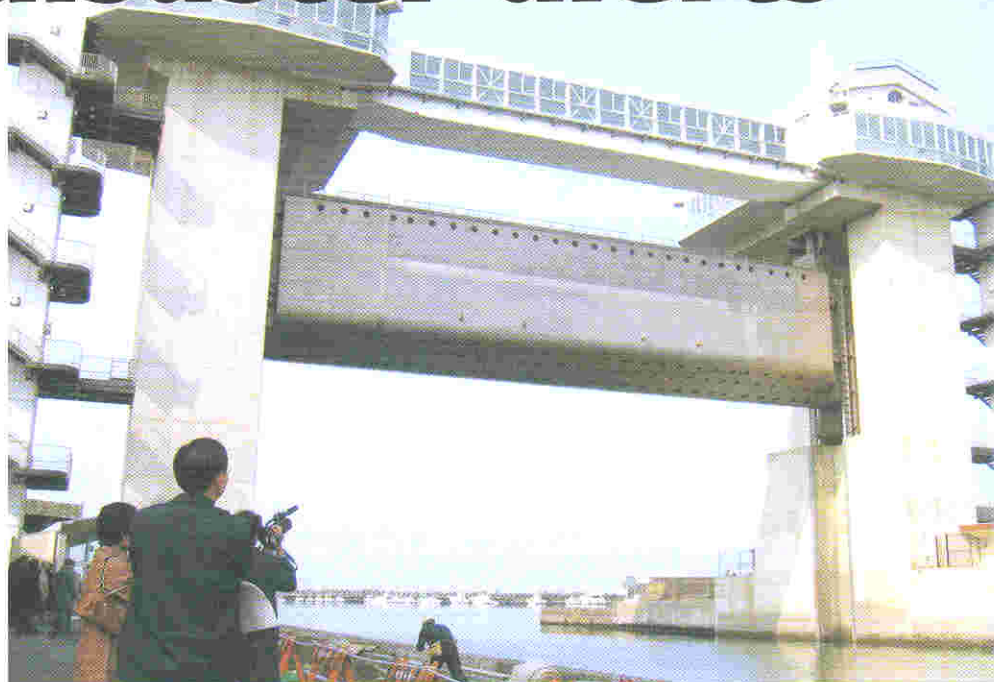
A tsunami floodgate in Shizuoka in central Japan
